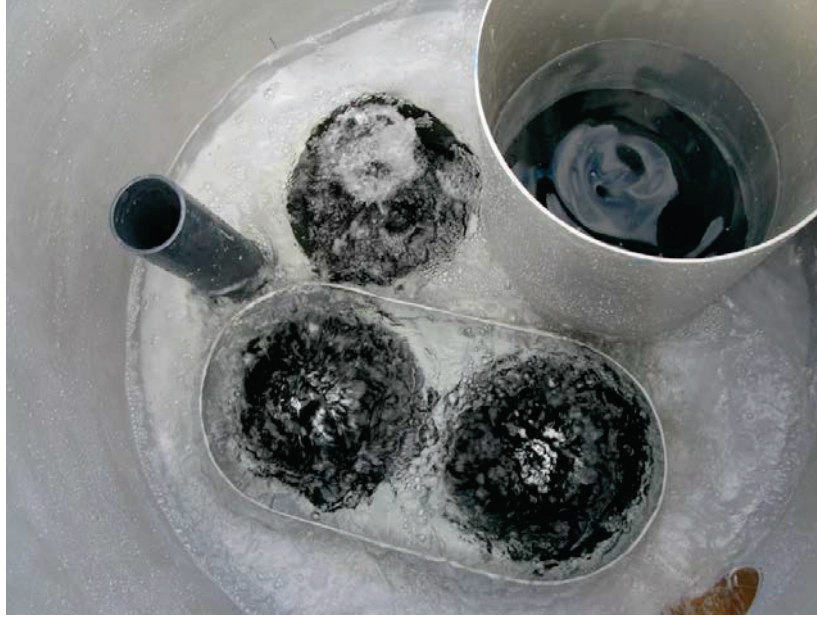
Figure 8 Top view photo of the Jellyfish® Filter JF4-2-1 during operation. Filtered water exits the cartridge lid orifice as a pulsating fountain.
