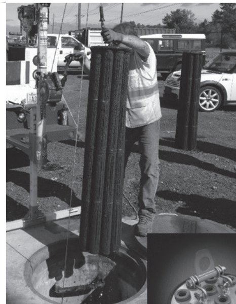
Cartridge Removal & Lifting Device
