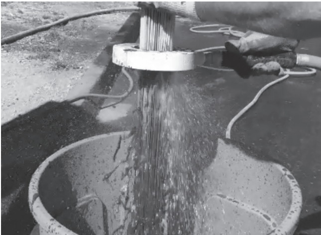
Vacuuming Sump Through MAW
