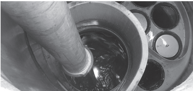
Vacuuming Sump Through MAW
